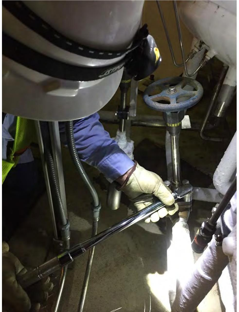
**Reassembly of BK9412T applying proper torque with torque wrench**
